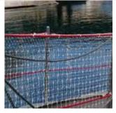
Applied and fixed on handrails (rope 16mm) Square 50 x 50 mm – safety net rope around the perimeter Lenght : 1m x 10m
